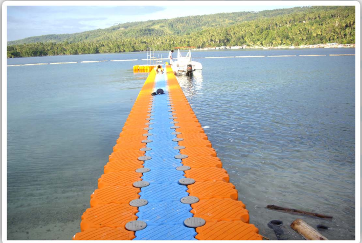
■ PONTOON BRIDGE Pearl Farm Davao
